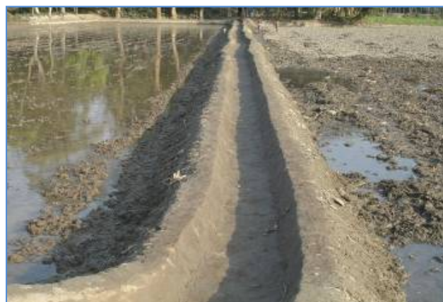
Photograph 1. Improve earthen irrigation channel
